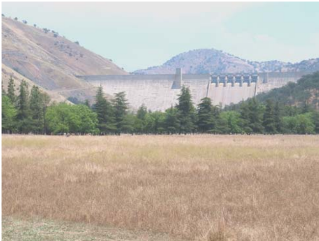
Pine Flat Dam
